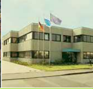
STOCKO Headquarters in Wuppertal
