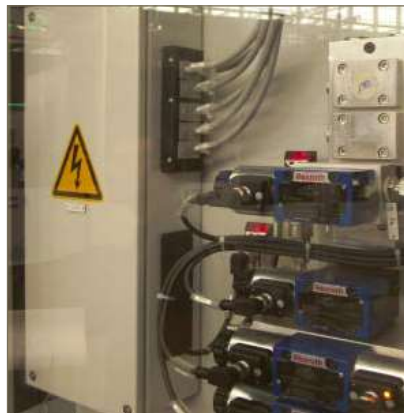
KEL 24|10 - Page 16 / BPK 24 - Page 154 Routing of 6 cables with one cable entry frame. Another cut-out is sealed by a plastic blind plate BPK 24.
