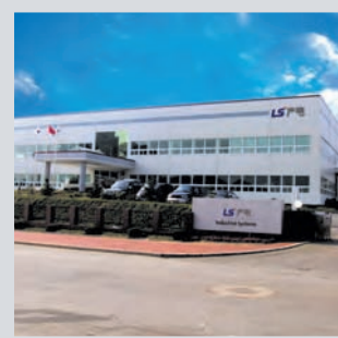
Dalian Plant (China)
