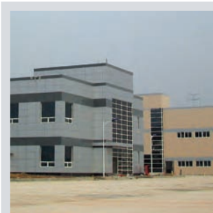
Wuxi Plant (China)
